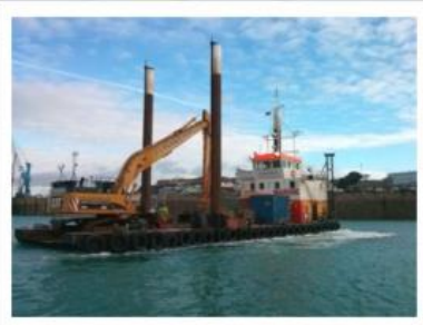
Dredging & Marine Construction
